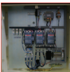
Star delta starter. Soft start is optional.
