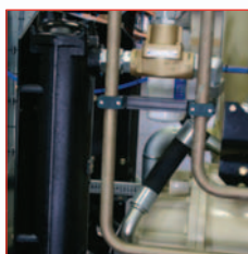
Sea water coolers. Shell and tube facilitates cleaning.
